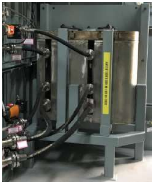
Fig. 4a. TCCR Filter Housings & Shield Assembly
