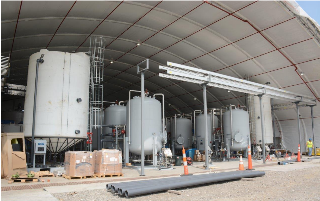
Figure 5. C- and D-Trains
