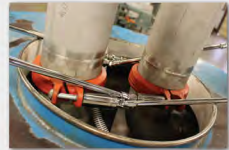
SCF™ Liner Piping Victaulics with ALARA Extensions
